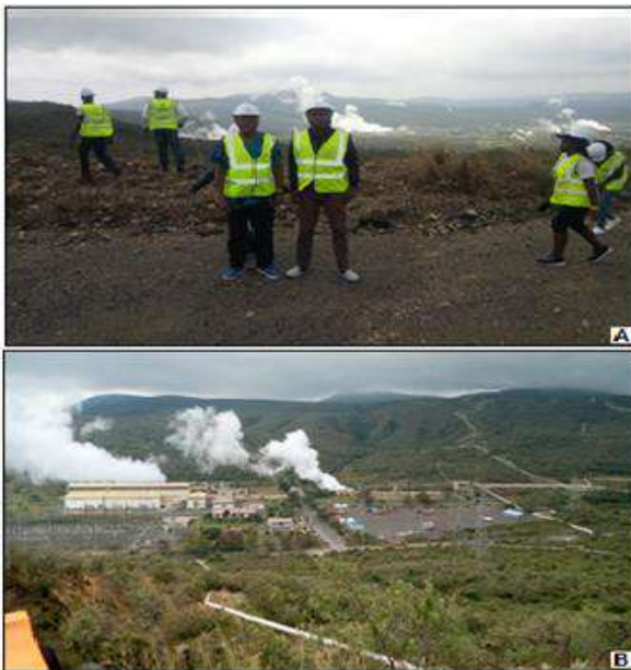
Figure 16: Above Olkaria Geothermal Plant System and geysers (A) and (B)
