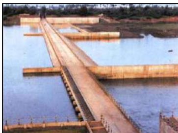
Fig -4: Photo of weir constructed on Tapti River
